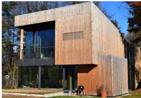
Fig. 1 – Facade of the SSH.
