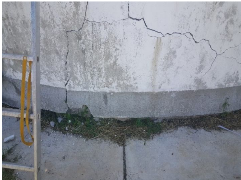
Fig. 1 – Crack in the outer wall of the water tank.
