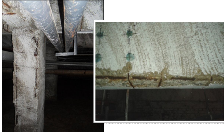
Fig. 6 – Structural elements degradation due to poor maintenance at the water system.
