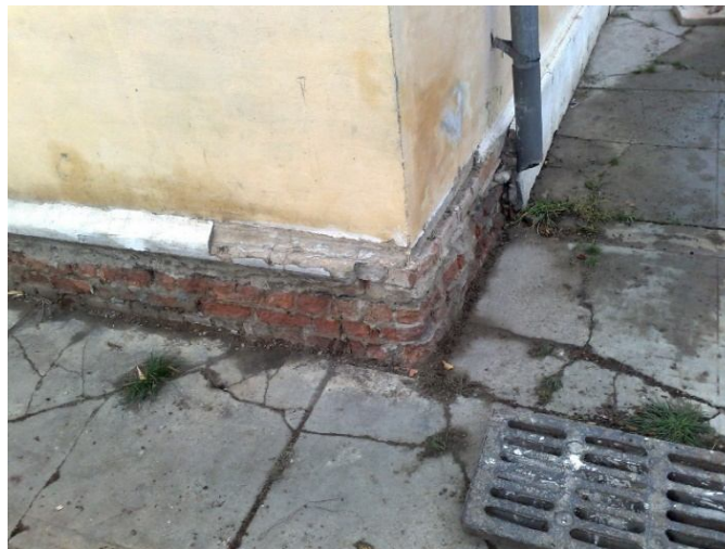
Fig. 4 – Sidewalks degradation allowing water infiltration.
