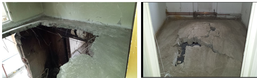
Fig. 8 – Explosion effect due to gas seepage.
