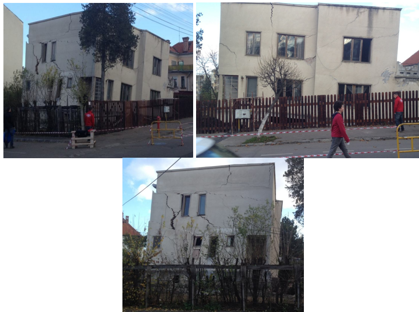
Fig. 5 – Damaged house due to problems at the foundation soil level.
