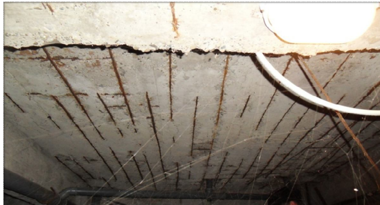
Fig. 7 – Extensive reinforcement corrosion of the slab over a technical basement due to water and chemical seepage.
