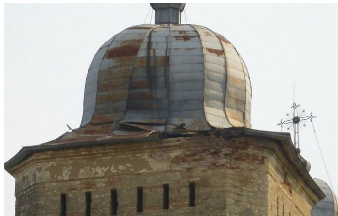
Fig. 2 – Damaged roof of a historical building.
