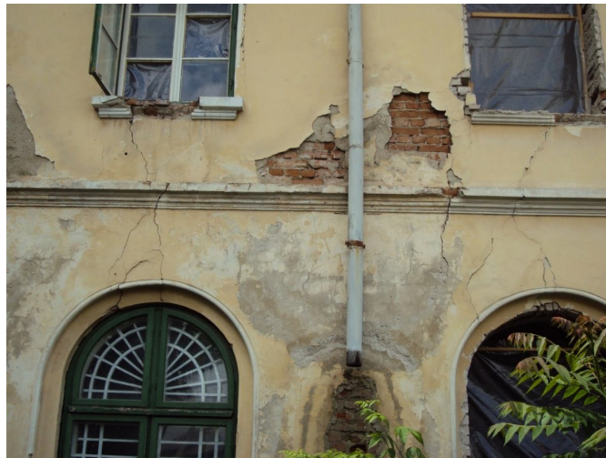
Fig. 3 – Exterior damage of a historical monument due to rainwater leakage.
