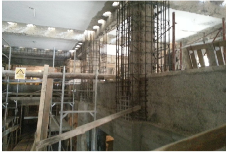
Fig. 3 – Concrete jacketing of columns, plates and walls.
