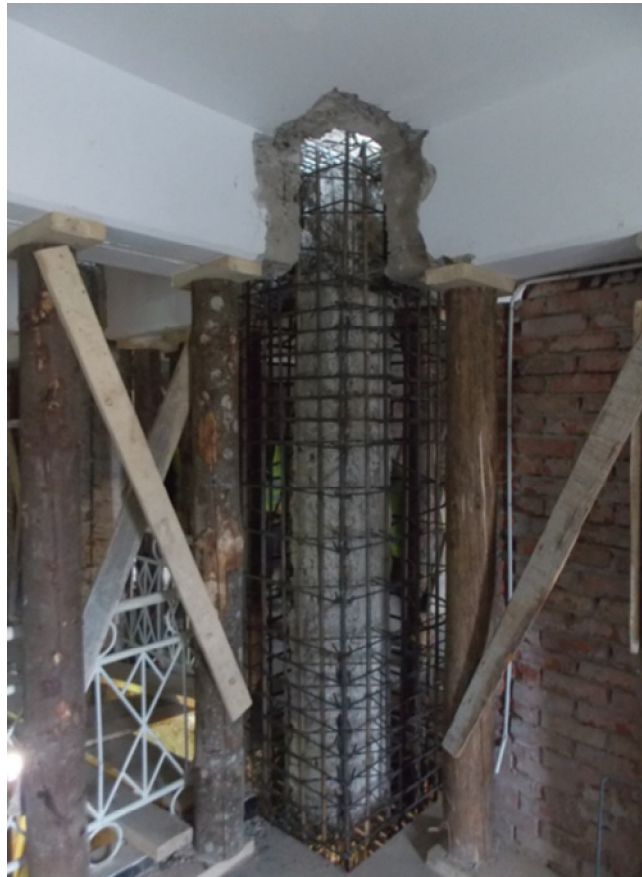
Fig. 5 – Reinforced column. Note the damage done to the paintwork.
