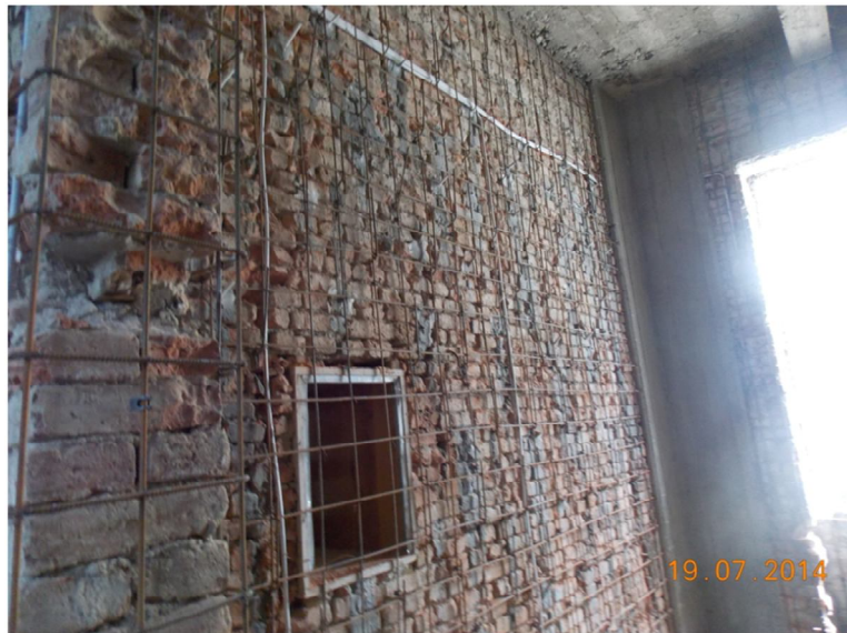
Fig. 4 – “New” wall reinforcing, ready for formwork and casting.
