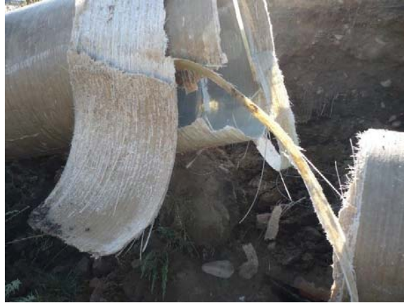
Fig. 2 – Fault in land contaminated with oil Dărmănești/Bacău, Romania.
