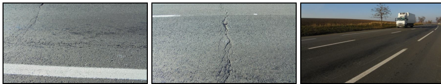
Fig. 3 – Distresses on Sample E2.
