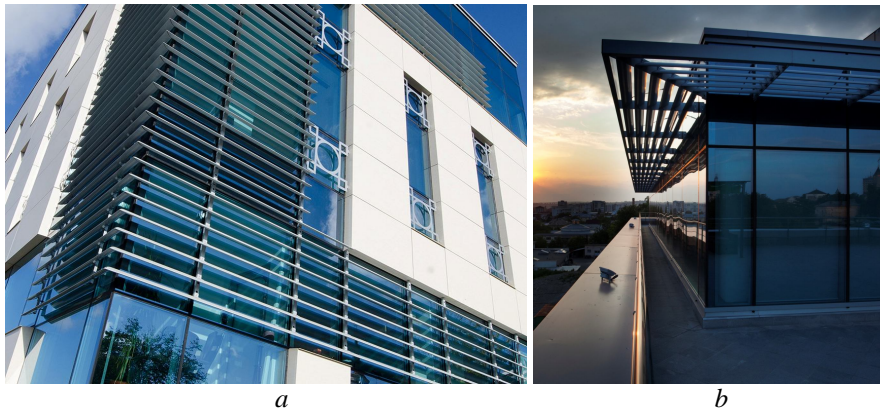
Fig. 3 – a – fixed brise-soleil on the South-Eastern and South-Western façades; b – cantilever shading element at last level.
