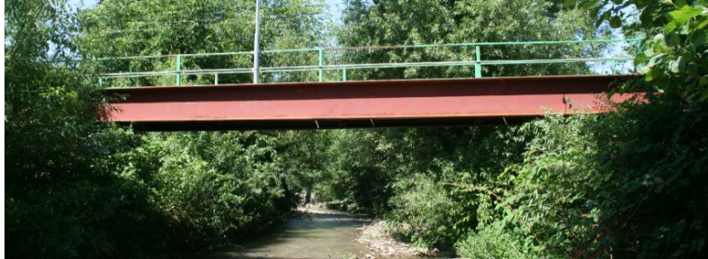
Fig. 4 – Footbridge built in Bihor County.
