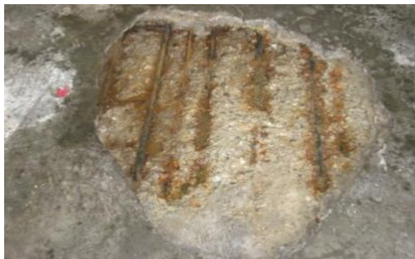
Fig. 9 – Carbonated concrete.
