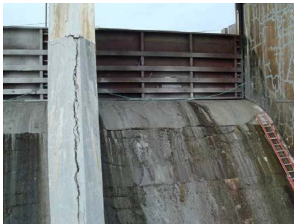
Fig. 12 – Alkali-aggregate reaction.
