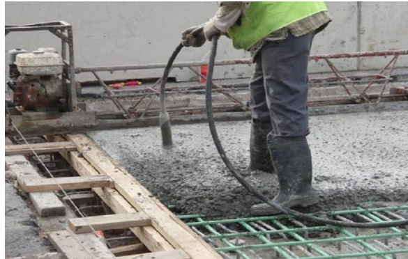
Fig. 4 – Compacting fresh concrete.
