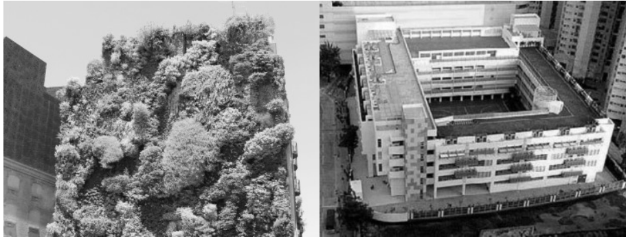
Fig. 1 – Left: Green walls system - Continuous living wall system, Caixa Forum, Madrid, June 2013 (picture taken from Manso & Castro-Gomes, 2015). Right: Primary School at Sze Mei St, Ho Man Tin (picture taken from Zhang et al. , 2012).
