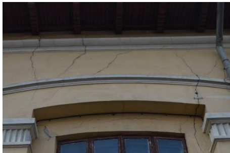
Fig. 12 – Vertical cracks in masonry parament.
