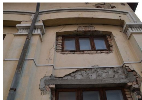
Fig. 11 – Fissures over the lintels (where are present).
