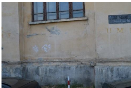
Fig. 20 – Infiltrations of water to the socle.
