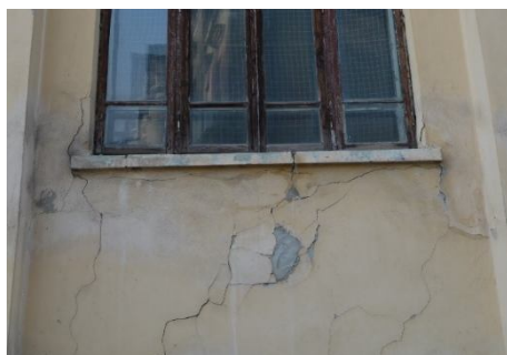
Fig. 10 – Inclined cracks on the masonry wall.
