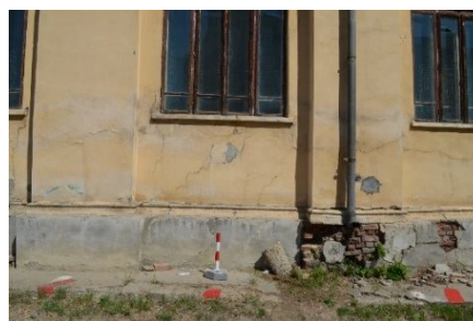
Fig. 15 – Crushes and breakdowns of the socle bricks.
