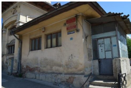
Fig. 16 – The annex building (without seismic joints).
