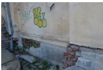
Fig. 14 – Detachments of the socle.
