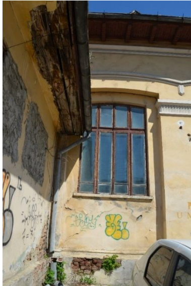
Fig. 18 – Water infiltrations in the straw.
