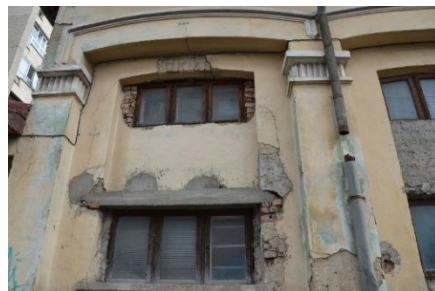
Fig. 21 – Rainwater infiltration.
