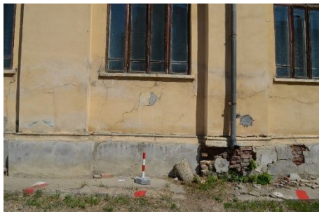
Fig. 22 – Settled and non-waterproof sideboards.
