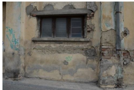
Fig. 17 – Non-compliant attempts to embed the lintels.
