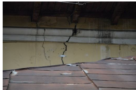
Fig. 23 – Major cracks under the roof.
