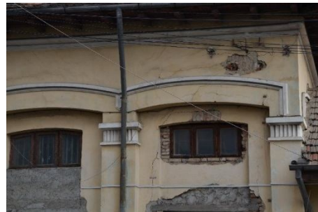
Fig. 13 – Plaster detachments.
