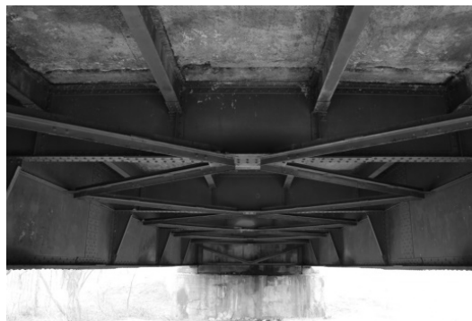
Fig. 4 – View of the bracing system.
