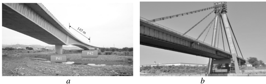
Fig. 1 – a – Caohu Bridge (Taiwan) (Sung et al. , 2016); b – Agigea Bridge (Romania).
