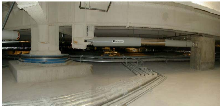
Fig. 9 – An example of viscoelastic damper (Morgan & Mahin, 2011).
