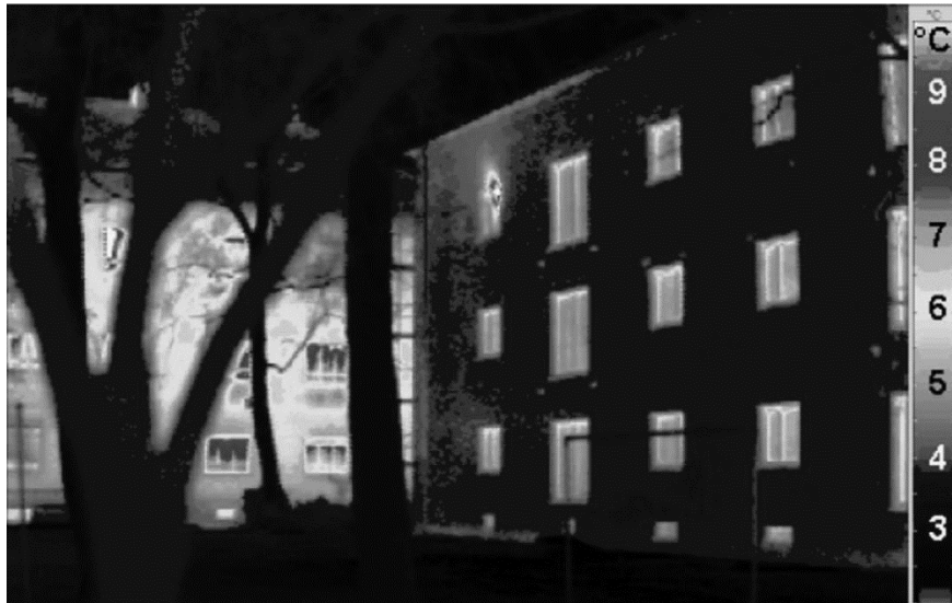
Fig. 1 – Comparison between Passive House (right: with a high level of thermal insulation) and a traditional building (left: with considerable more heat losses compared to the Passive House building). Infrared temperature measurements (Feist, 2002; Yang et al. , 2017).
