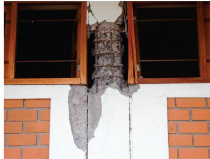
Fig. 7 – Damage to structural column (“captive column”) due to restraint caused by partial height masonry wall in the 2001 Peru Earthquake.
