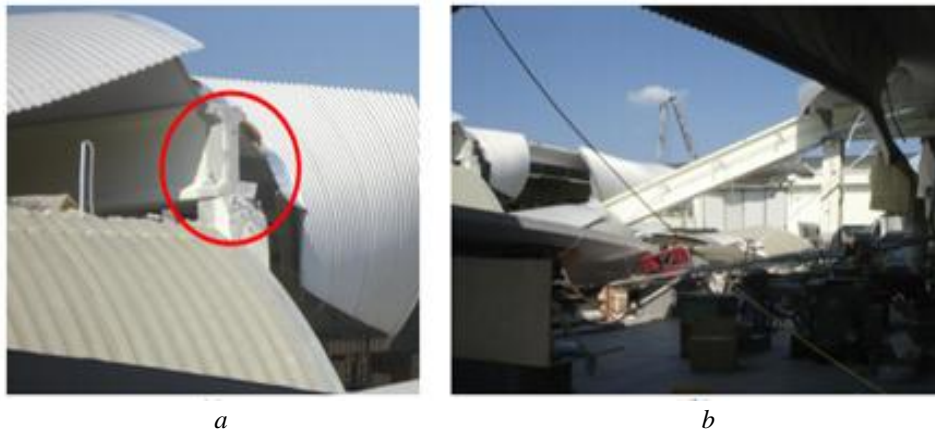
Fig. 1 – Failed precast connections (Magliulo et al. , 2014); a – Dowel beam-to-column connection failure and b – consequent loss of support of the beam from column.
