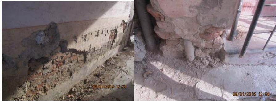
Fig. 5 – Destroyed masonry.
