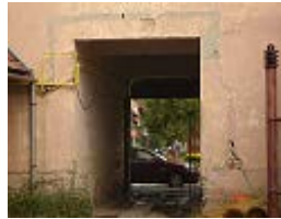
Fig. 2 – Access to the inner court through the corridor.
