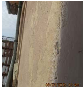
Fig. 4 – Degraded plastering.
