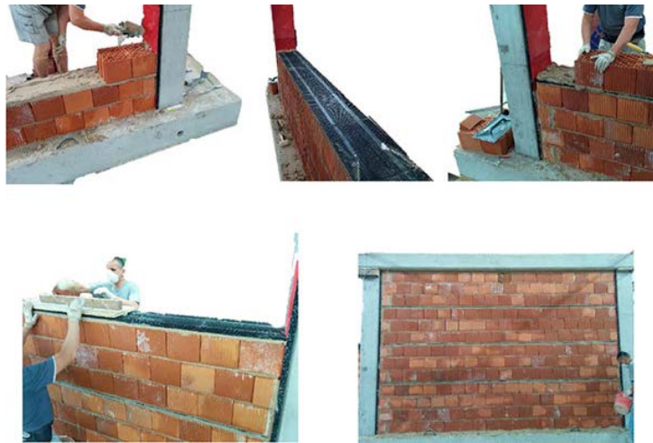
Fig. 4 – Masonry panel with rubber joint placed on perimeter and along the masonry rows.
