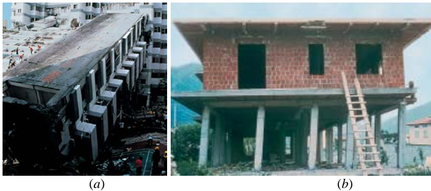
Fig. 6 – (a) Collapsed block of flats due to the ground floor columns failure (Taiwan, 1999); (b) Ground floor failure mechanism (Italy, 1976).
