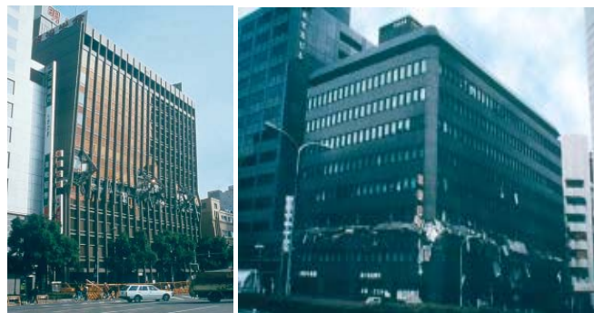
Fig. 7 – Examples of damaged structures due to an intermediate soft story (Japan, 1995).
