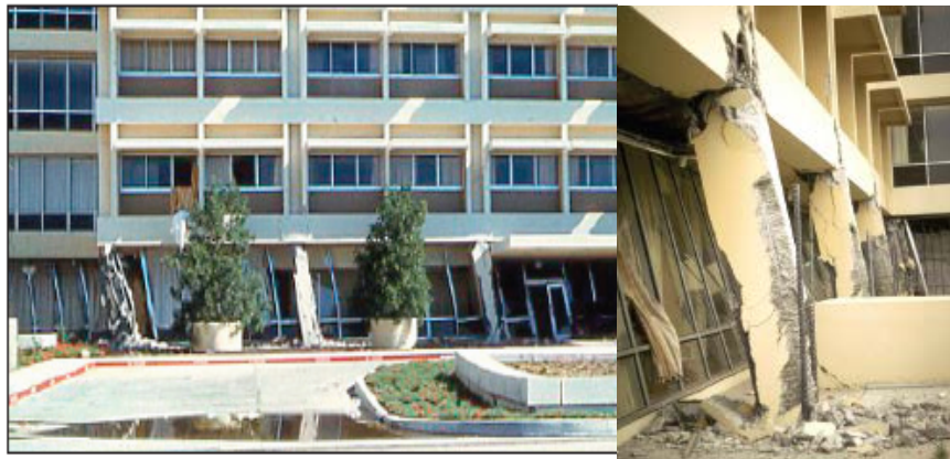
Fig. 9 – Ground floor failure mechanism of Olive View Hospital (San Fernando, California, 1971).
