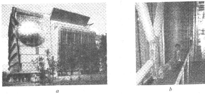
Fig. 6.- *a* - External view of building; *b* - view of a couple of dampers implemented.
