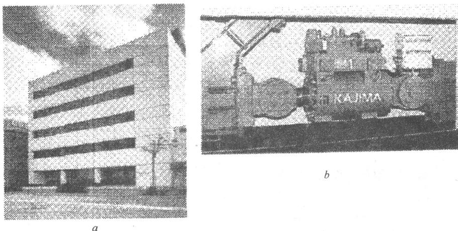
Fig. 5.- *a* - External view of Kajima Shizuoka Building; *b* - view of semi-active hydraulic damper.
