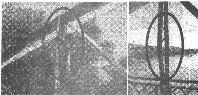
Fig. 2.- Degradations of the structural elements due to the impact with vehicles.
