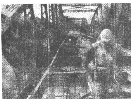
Fig. 26.- Sand blasting of the structure.
