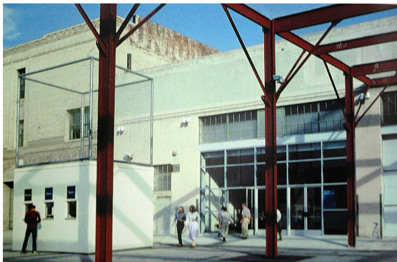
Fig. 2 – Contemporary Temporary Museum, Los Angeles, USA.
